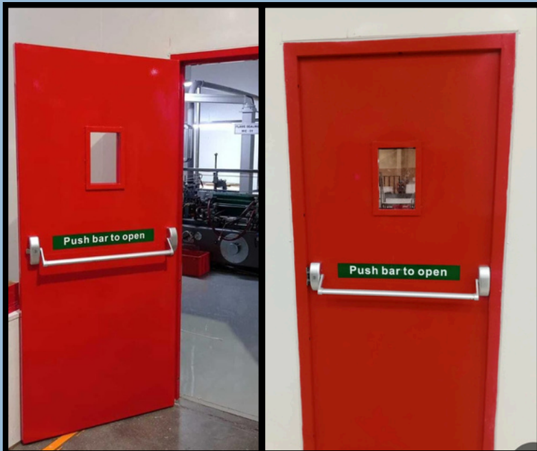
EMERGENCY EXIT DOORS
